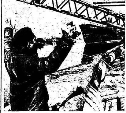
wide-gauge pipe containing a number of telephone cables was laid across the bottom of the Kishon Harbour by workers of the Communications Ministry yesterday. Divers and giant cranes were used in the operation, which is one of the first of its kind in the world, the Ministry claims. The new cable will be able to handle up to 2,000 calls from the north of the country to the central region, and will increase present capacity by 600 per cent.
